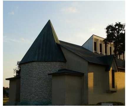
Giddings School, Giddings TX Architect - Edward Mattingly Associates Installed 1972
