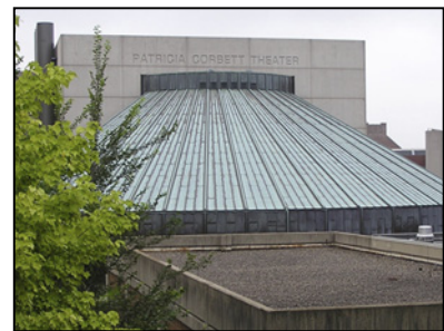
Patricia Corbett Theater, University of Cincinnati, CopperPlus roof installed in 1971
